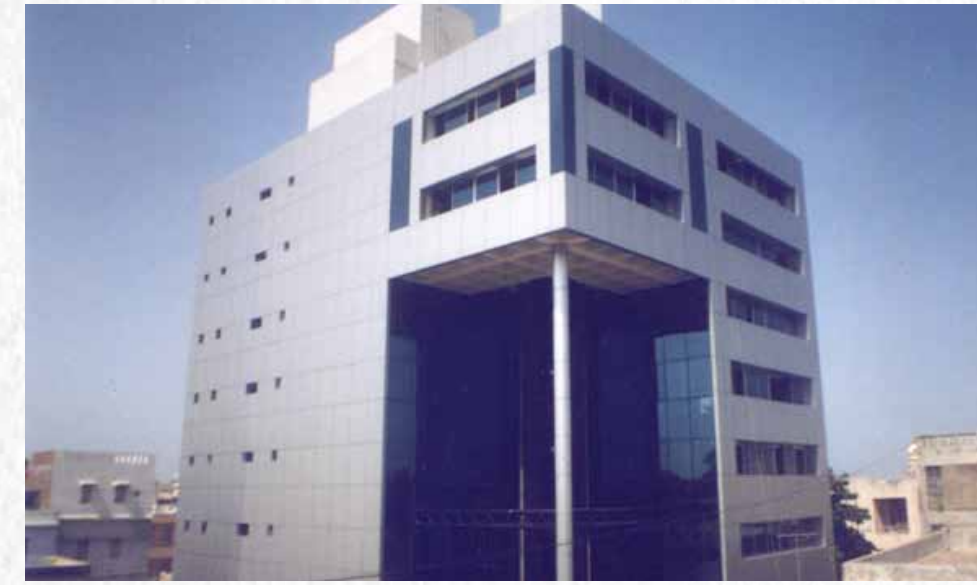
The Natpur Co-Operative Bank Ltd.
